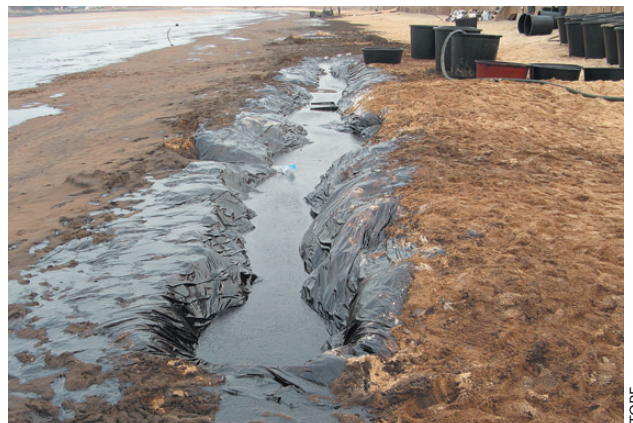
Use of a trench to recover oil
