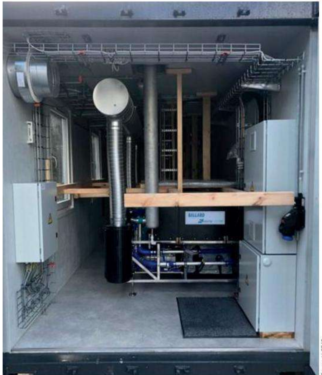
■ The installation of the Ballard HD-100 PEM fuel cells
