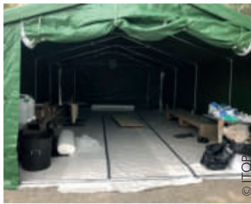
Example of worksite equipment
