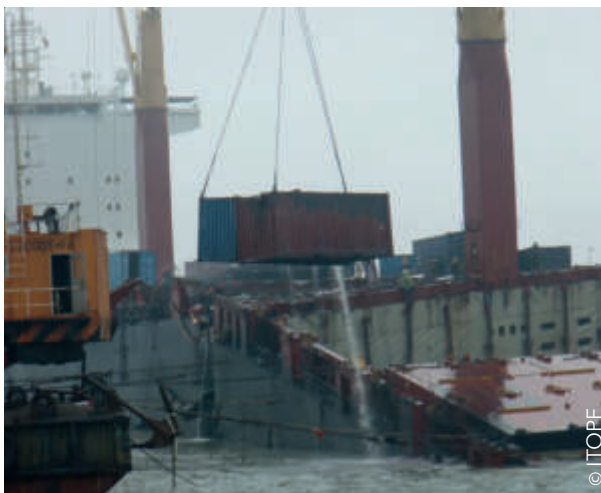
Recovery of collapsed containers
