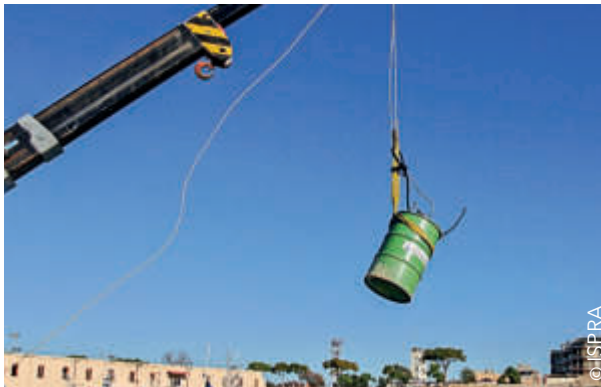
Lifting a drum with a crane
