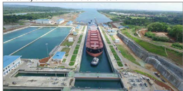
Test call of the new Panama Canal locks
