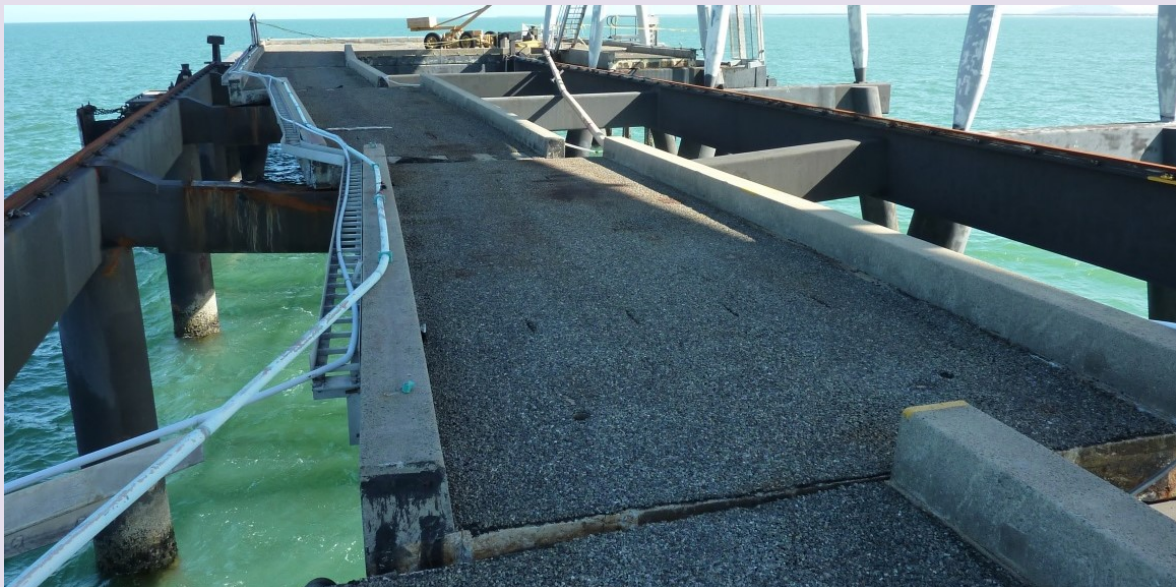
Box 21: Accommodating extremes in wharf repair design, Lucinda Bulk Sugar Terminal, Australia
