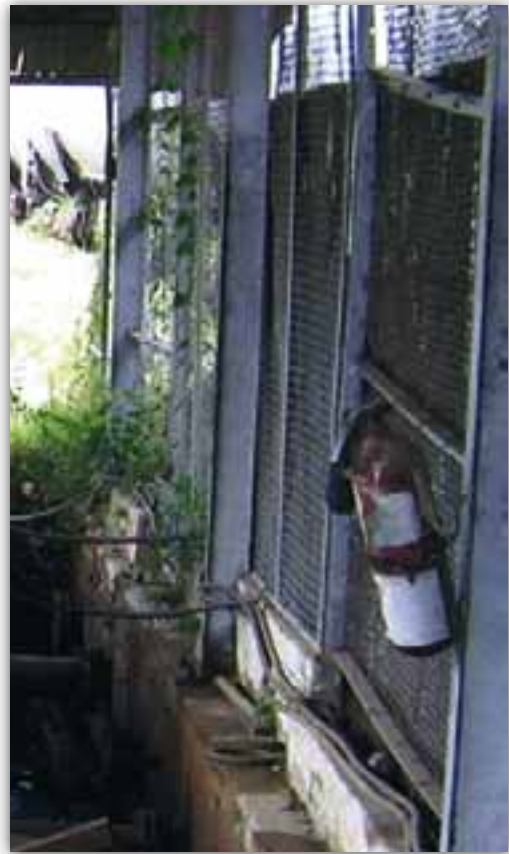
Figure 54: Fire Extinguishers in Poor Condition and Not Readily Accessible
