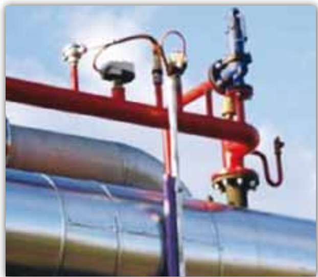
Figure 14: Pressure Relief Valve (painted blue)
