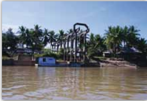
Concrete structure to hoist cargo between the train and at vessels at the upstream port on Don Deth
