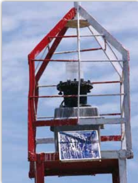
Solar panels from buoys (left) are supposed to recharge batteries during the day. But they are often stained by bird droppings and no longer working. The “safe water” buoy (right) seems to be a favourite gathering place for birds.
