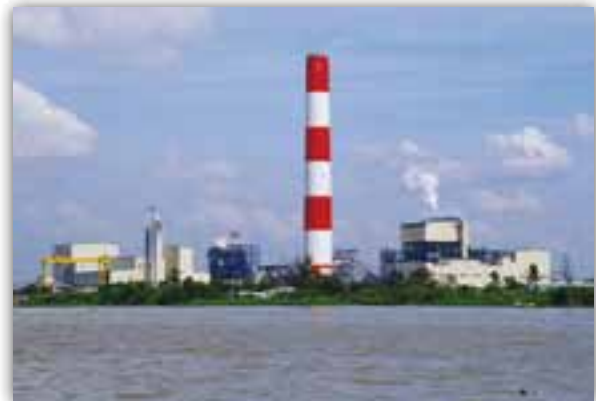
There are many ports and terminals on the right bank of the river between the O Mon River mouth and Can Tho. Most activities, however, are mid-channel.
