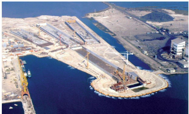
Figure 21. Hydrolift during the construction.
