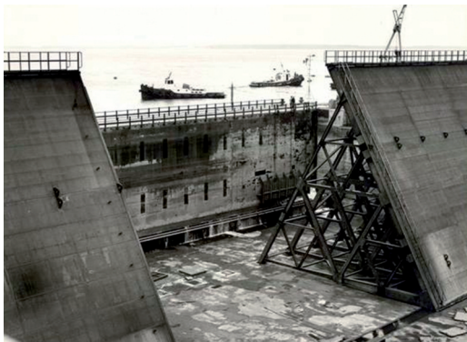
Figure 12. Mitrena shipyard - Gates in the entrance of dock 21.
