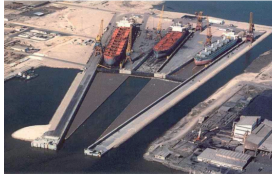
Figure 6. Hydrolift in the Mitrena shipyard.
