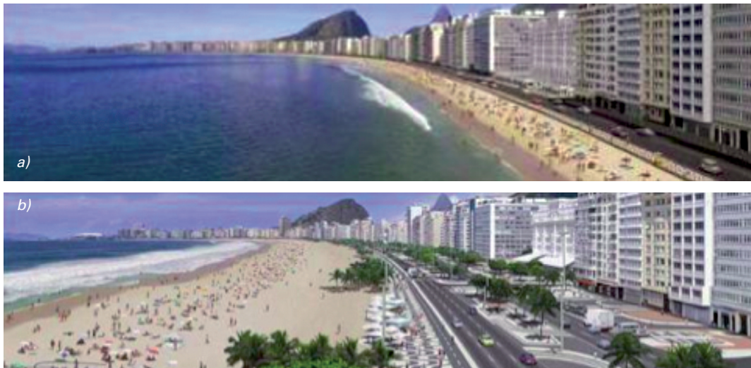
Figure 5. a) Copacabana beach in 1956; b) Copacabana beach after the widening in 90m with artificial nourishment. Studies and design of LNEC between 1968-1971.
