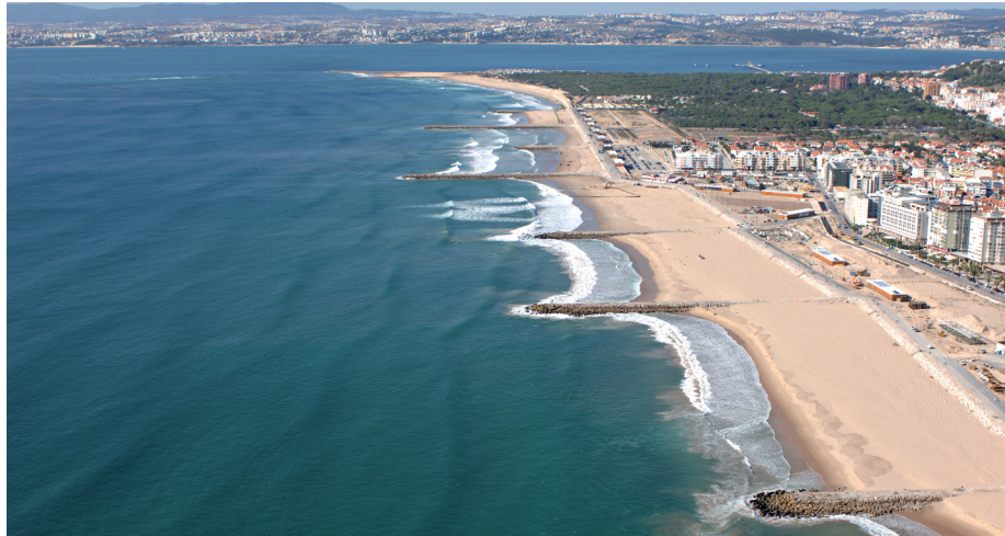
Figure 3. Groin field, seawall and artificial beach nourishment at Costa da Caparica.
